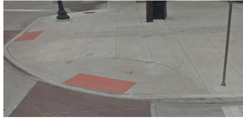
Sawcut Concrete Sidewalk
